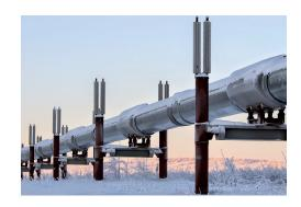
BACKGROUND Oil pipelines in Alaska can reach elevations of more than 4,739 feet and encounter air temperatures as low as -95°F (-71°C). It's cold and inhospitable. And if the oil flow freezes at any point along that stretch, it could spell catastrophe for the pipeline operator. Thawing out pipes is a lengthy process that could be impossible in winter, when temperatures plummet in hard-to-reach locations.
